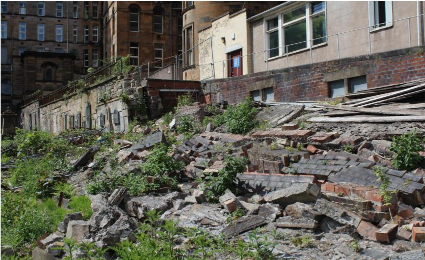
**Being the Restoration of the Fallen Section** - 20 metres of collapsed section of wall and walkway requires completely rebuilt.
