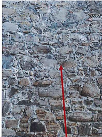
bulge area with minor crack
