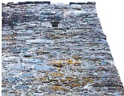
West wall with missing slate copes
