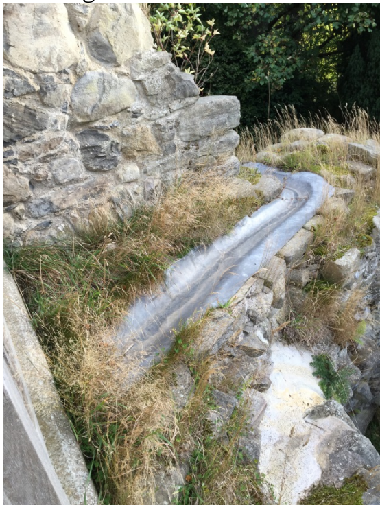
Lead gutter overgrown.
