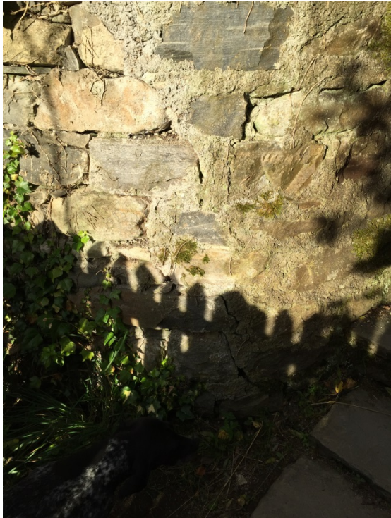
South east internal wall, bottom of staircase, Old Portland Cement visibly cracking.
