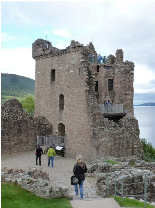
Photograph 2: Grant Tower looking from the south.
