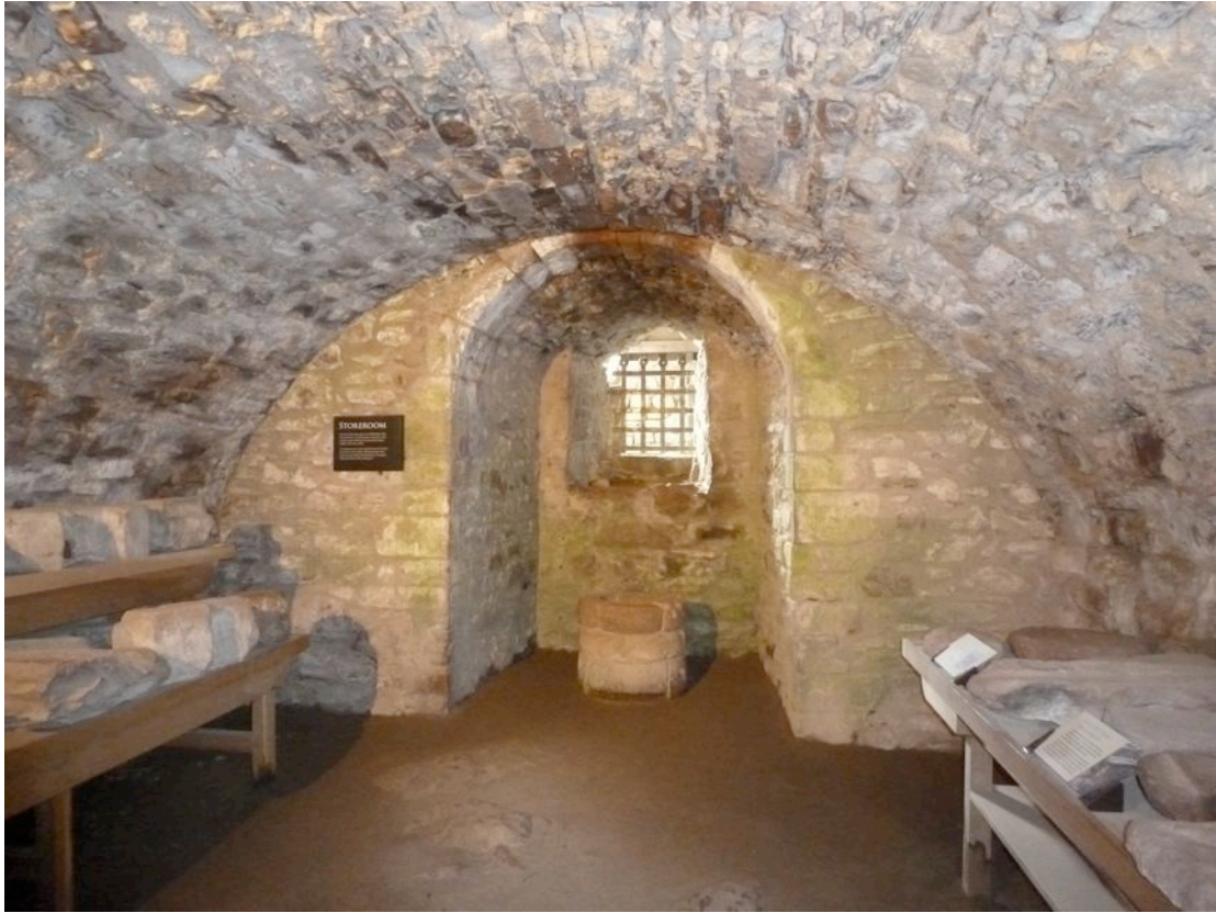
Photograph 5: The store room in the basement.
