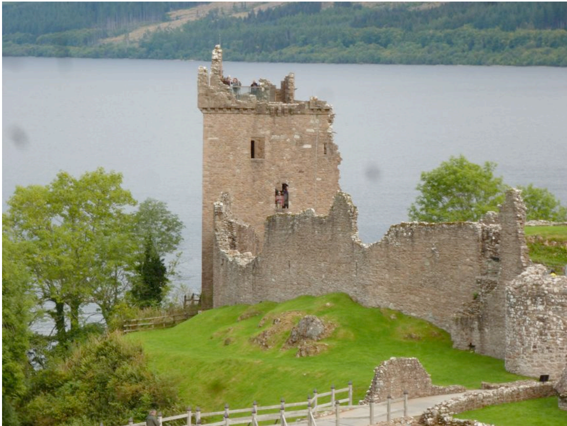
Photograph 1: Southwest face of the tower
