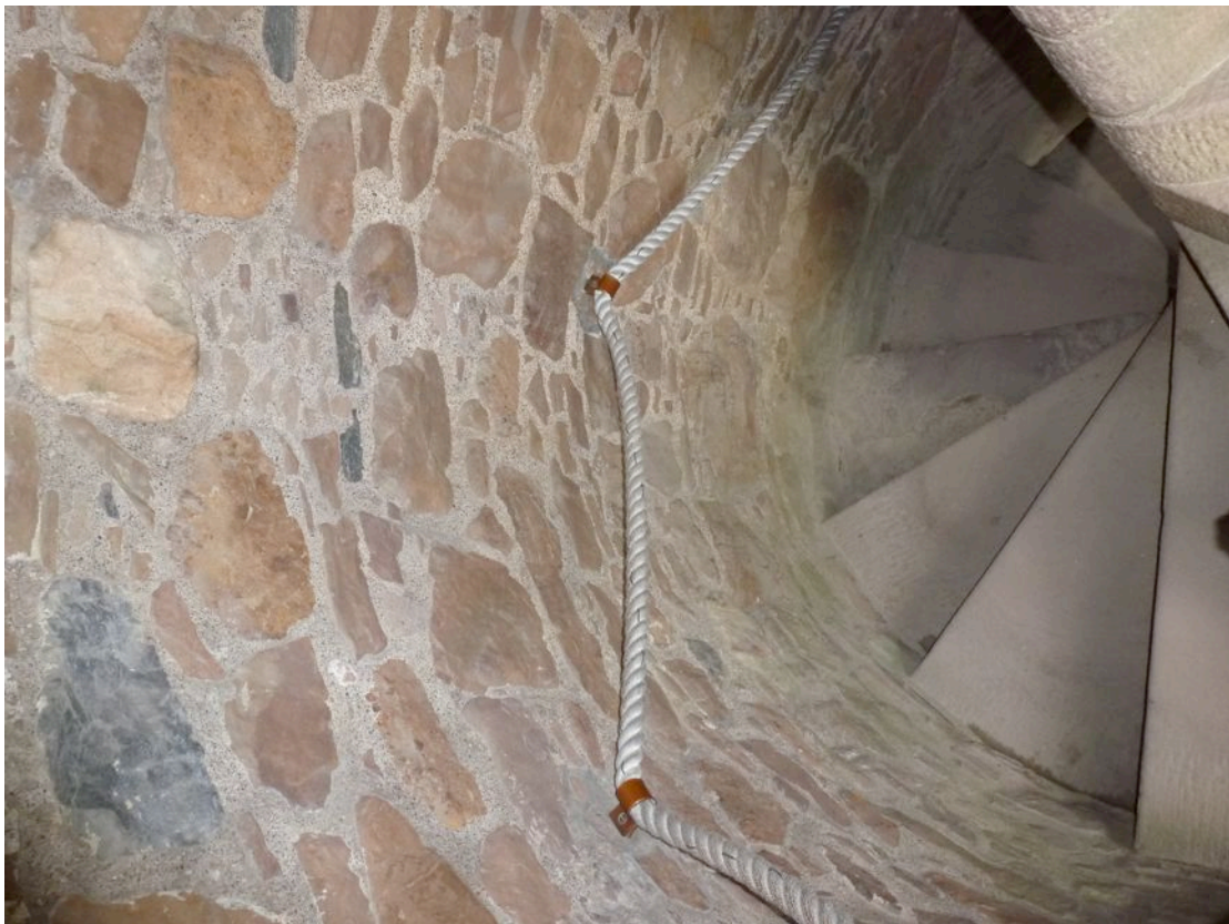
Photograph 6: The internal staircase.
