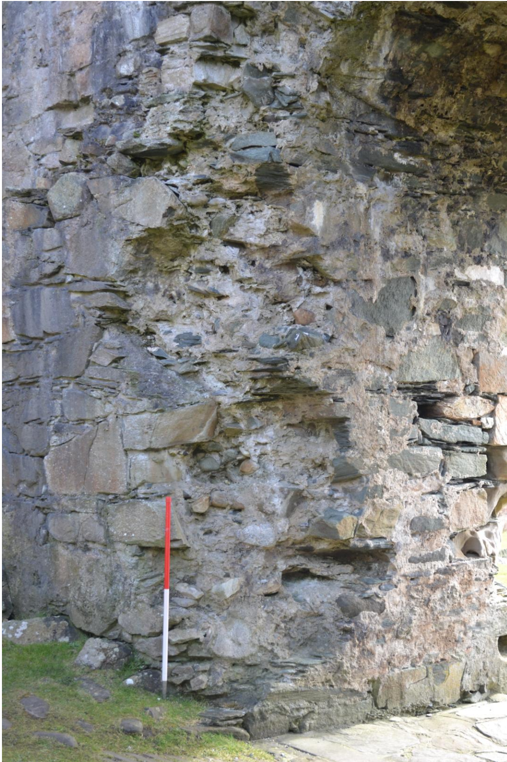
Figure 1 – A likely sample context at Castle Sween - exposed core at ground level.
